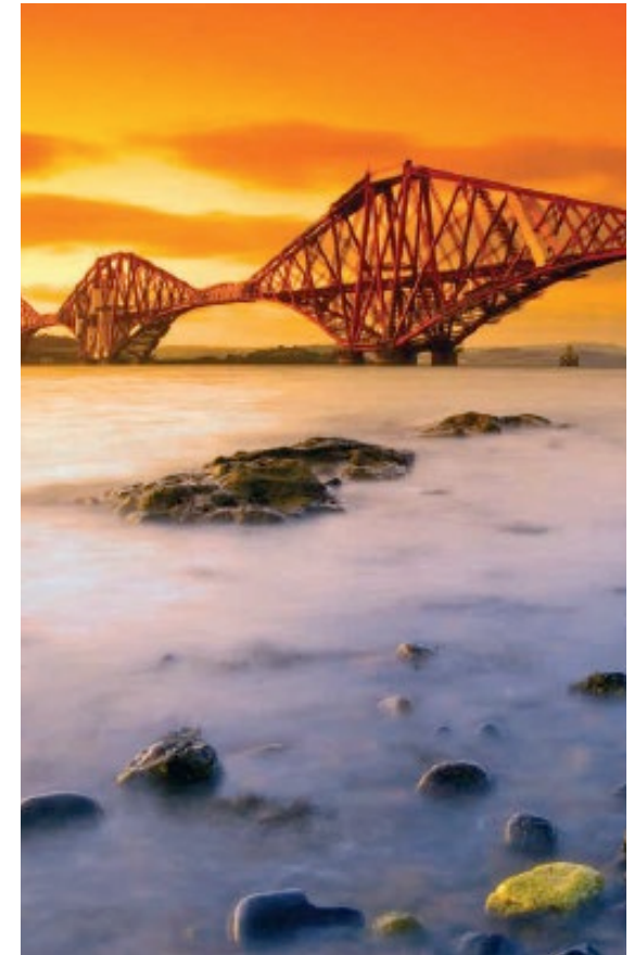
Forth Rail Bridge now 126 years since its completion in 1899 © George Gastin / Wikimedia Commons
