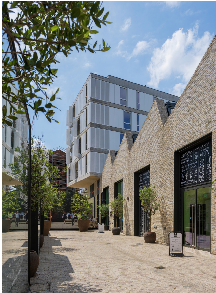
Rich Industrial Estate © London Square Developments Ltd
