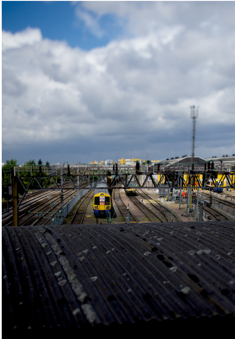
View of existing industrial and rail infrastructure at Old Oak © Matr Media
