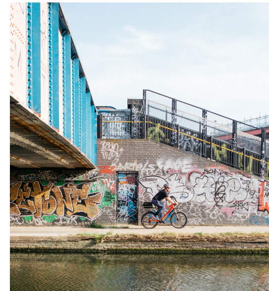
View of Mitre Bridge and the Grand Union Canal © Matr Media Ltd
