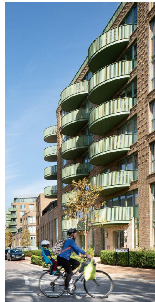
Meridian Gate, Kidbrooke Village © CZWG Architects
