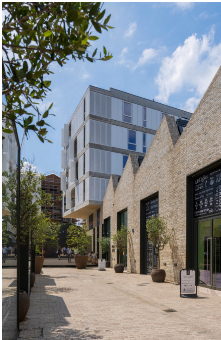
Rich Industrial Estate © London Square Developments Ltd
