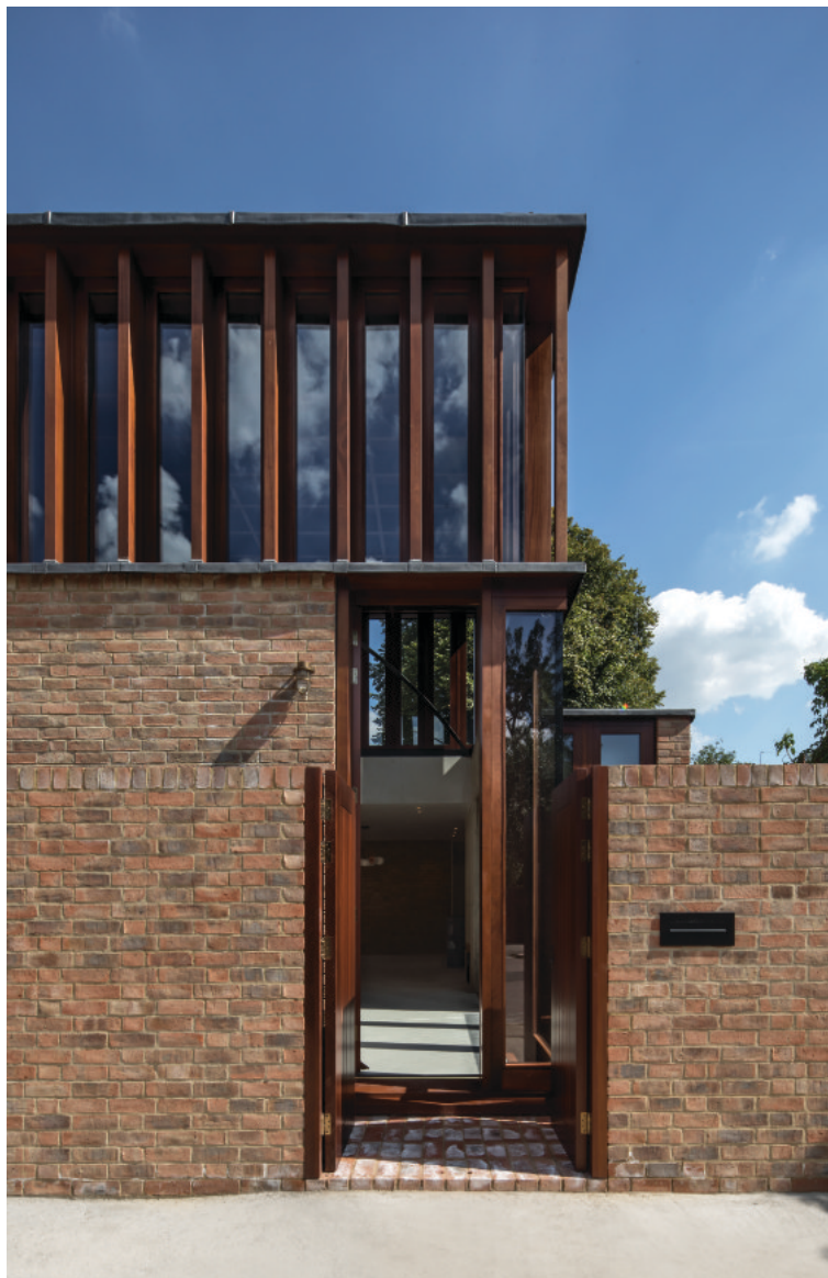
Periscope House, Woodville Road © Groves Natcheva
