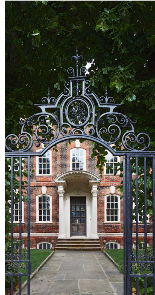
Gate at Rainham Hall, restoration, Julian Harrap Architects © Dennis Gilbert / Sue Salton
