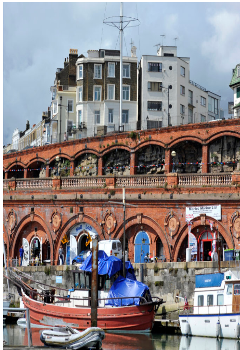
Royal Harbour Arches © Thanet District Council
